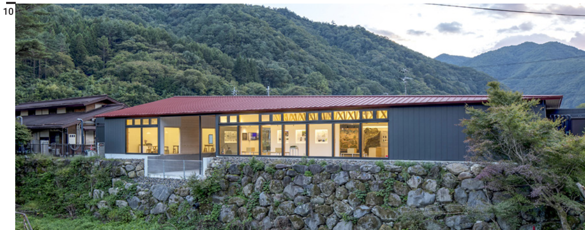
Fig. 10 Mt. Ontake visitor center Sato-terrace Mitake, yHa architects, 2022 (photo Takeshi Yamagishi).
