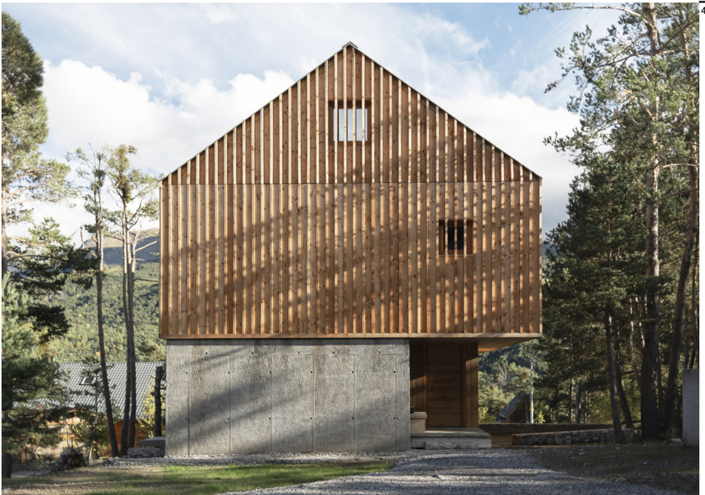
Fig. 4 External view of the North-West façade.
