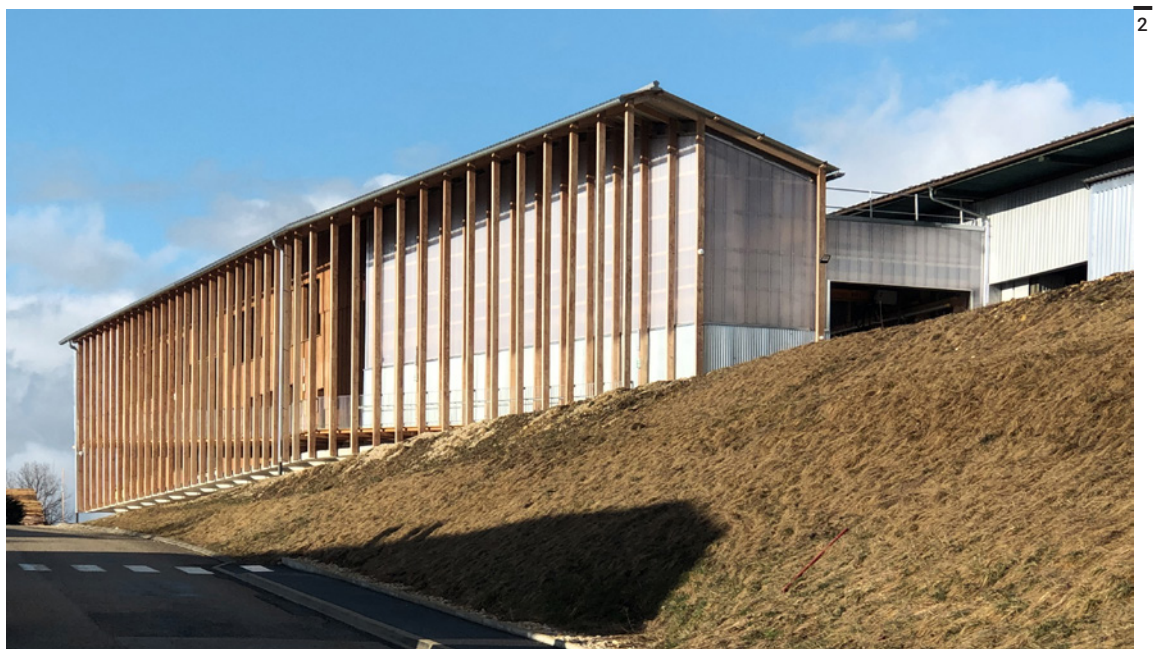
Fig. 1 Detailed external view of the roof structure.
