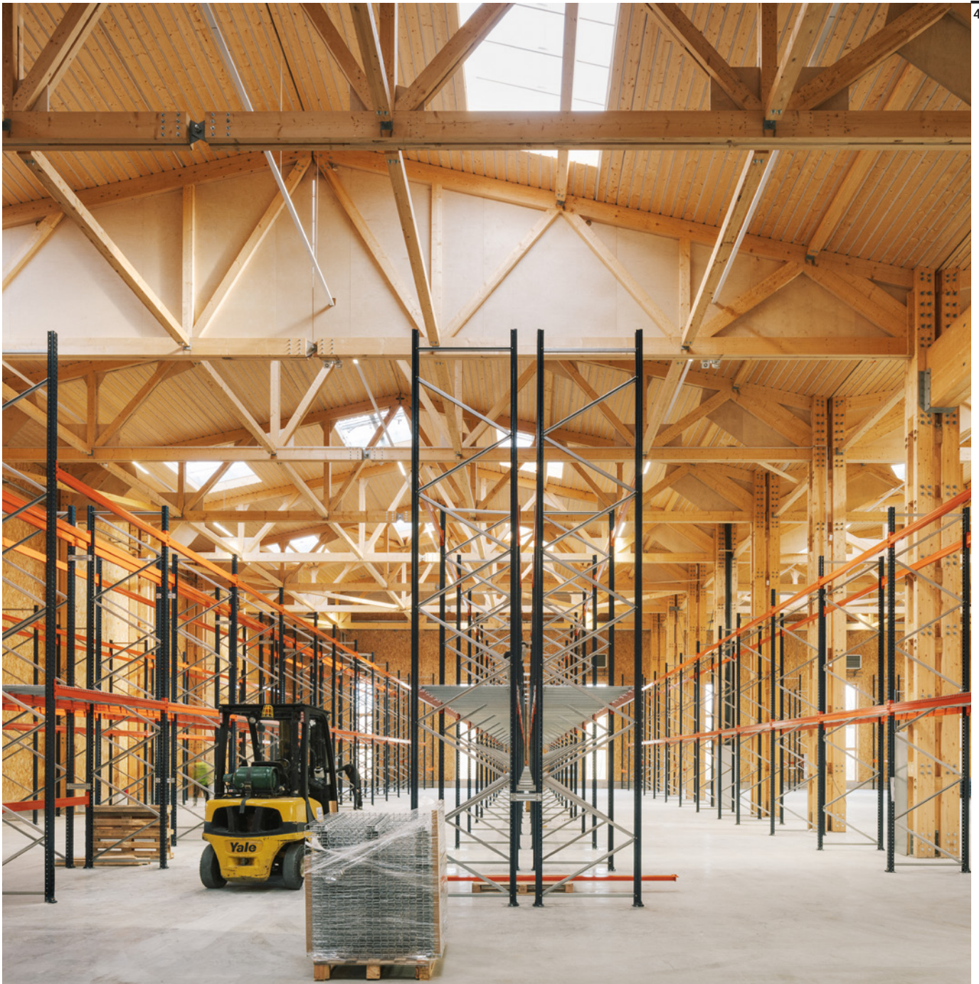
Fig. 4 Internal view of the warehouse.
