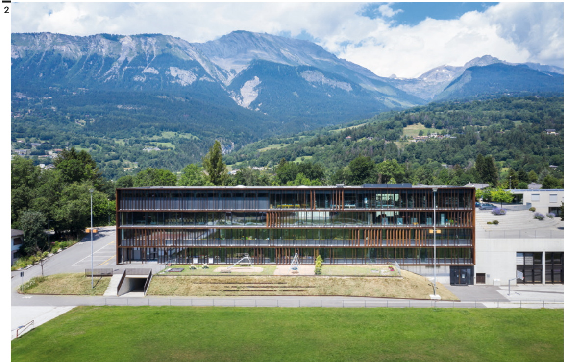
Fig. 1 External view of the West elevation.
