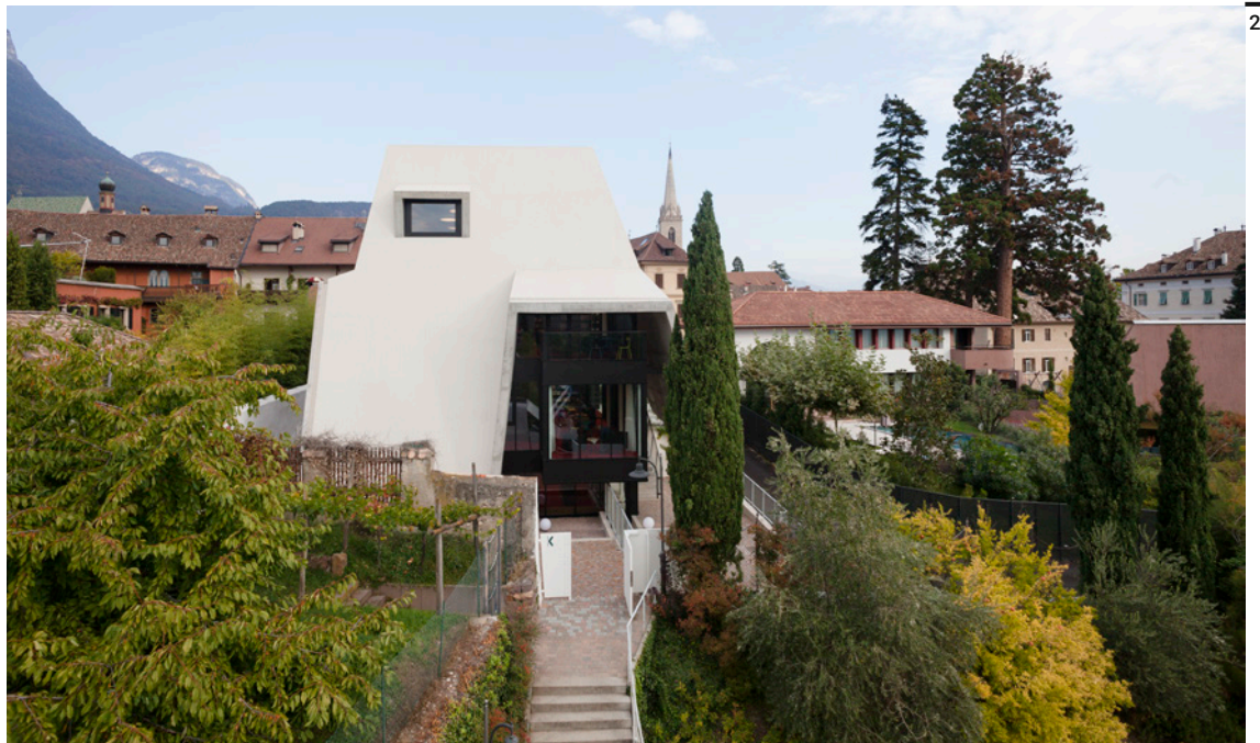
Fig. 1 External view of the North elevation.
